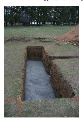
A more "finished" view of a guy anchor pit (filled with concrete)
