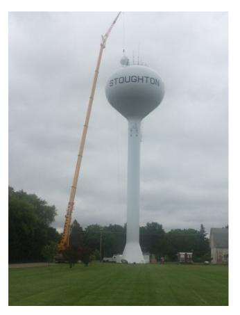
Microwave dish (antenna) being put in place on top of the Stoughton water tower. The dish is
